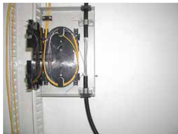
Figure 3 Splice Closure Converting Optical Fibre Ribbon into Pigtail
