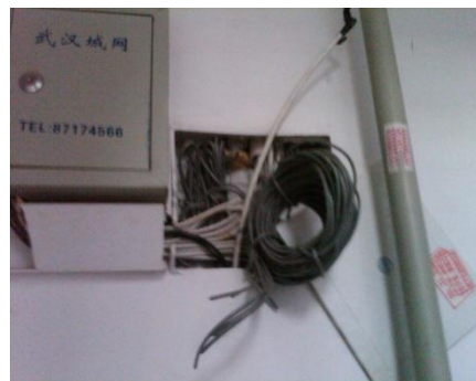
b. Distribution box on the third floor
