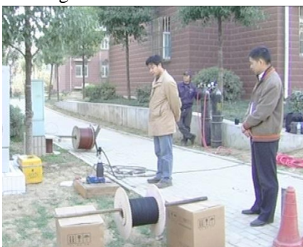
a. Air blowing optical fibre units
