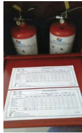
Checking and control of fire equipment
